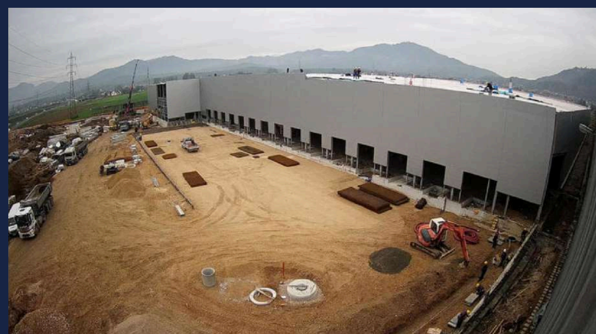
Labore in Kranj. The warehouse for DSV and Goodyear.
